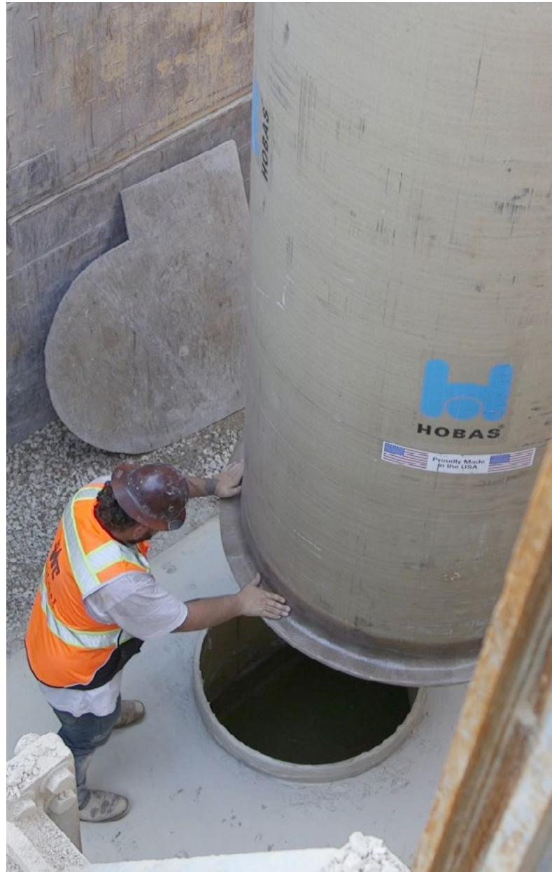
Manhole installation in Boise, Idaho.
