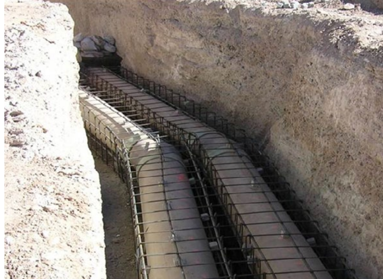
Axial concrete encasement
