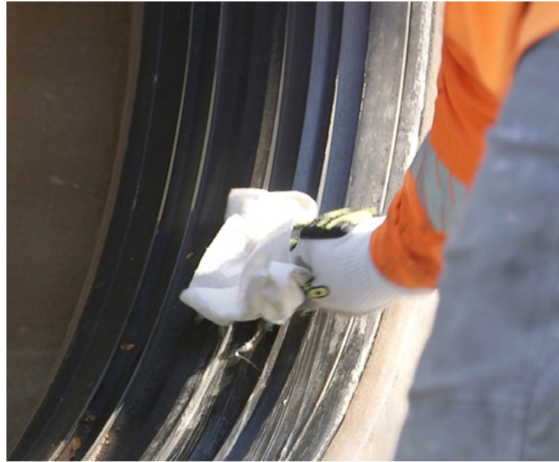
FRP coupling being prepped for installation
