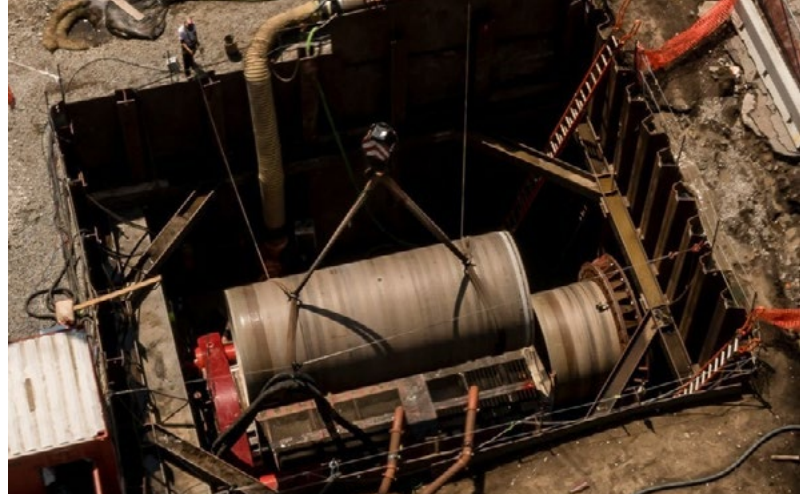
Jacking pipes have rubber ring sealed flush bell-spigot joints for quick assembly
