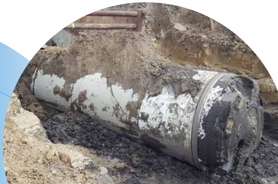
An Earth Pressure Balance Machine (EPBM) exits the Cliff Avenue crossing in Sioux Falls, South Dakota.
