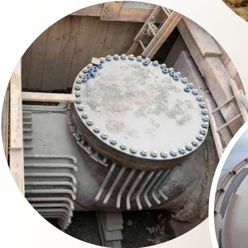
By pass structure
